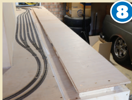
8 With the extension for the level fiddle yard in place the inclined section was fitted in place for the final time. 4.0 35mm screws were used throughout to secure it to the risers.
