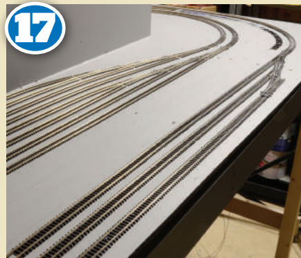
Plain track was then added to create the three through lines for the outer circuit storage tracks.
